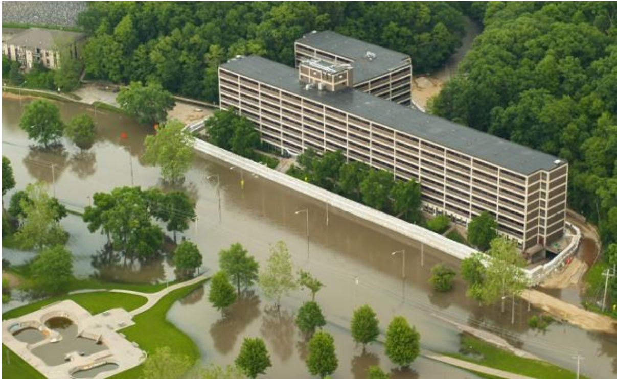
Fig. 1: Protection of the built up facility by adequate waterproofing of a boundary wall from flood inundation
