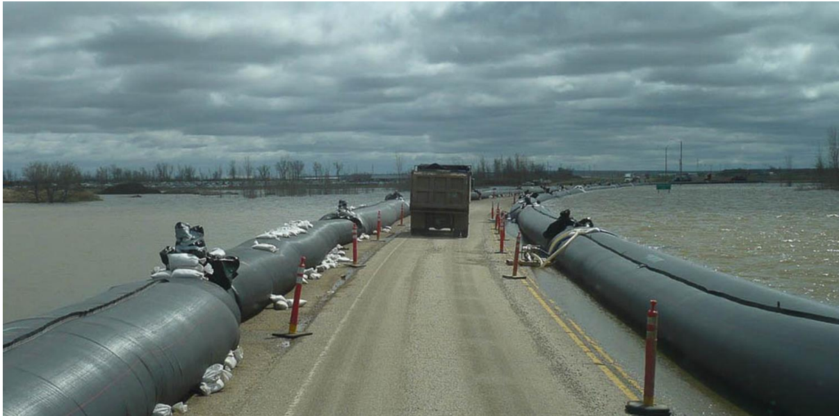
Fig. 3: Living with flood by AQUA Dam
